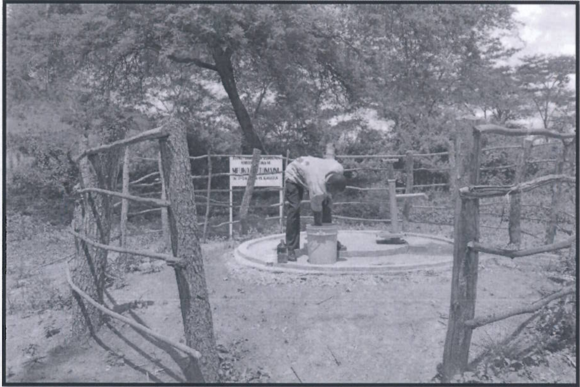
Figure 8: Tumaini worker cleaning the Tumaini-funded water pump for local village with chlorine (With permission of all persons in photographs).
